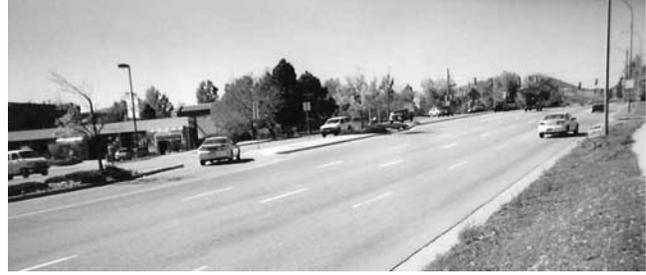
Figure 16. Directional median opening at three-leg intersection.
