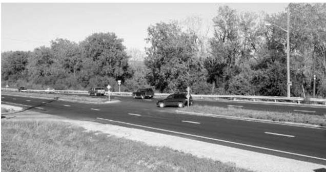
Figure 15. Conventional median opening at three-leg intersection.
